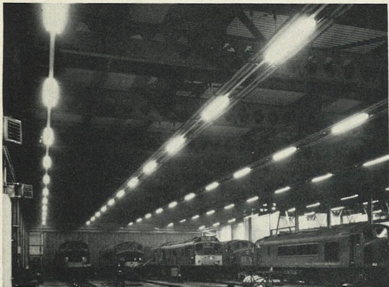
Toton Diesel Shed with integrated heating/lighting system.
