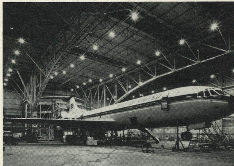
Hangar lighting at Gatwick with high bay fittings
