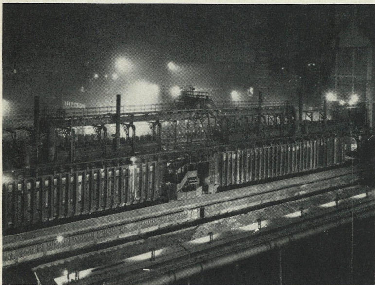
Coke ovens at Beckton lit by Atlas floodlights.
